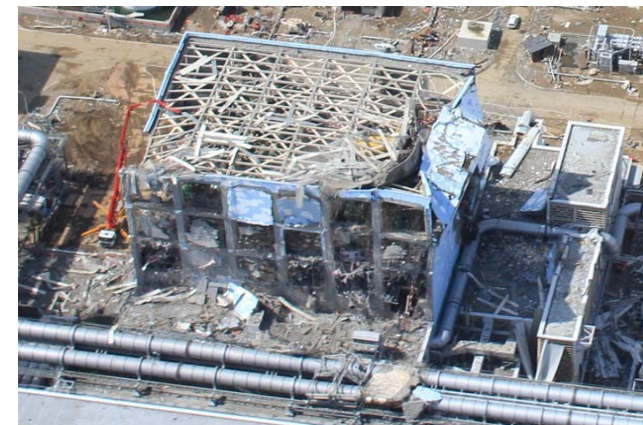
Reactor No. 4 (East side) Hydrogen built up in the 5 th & partially in the 4 th , floor (east west)
