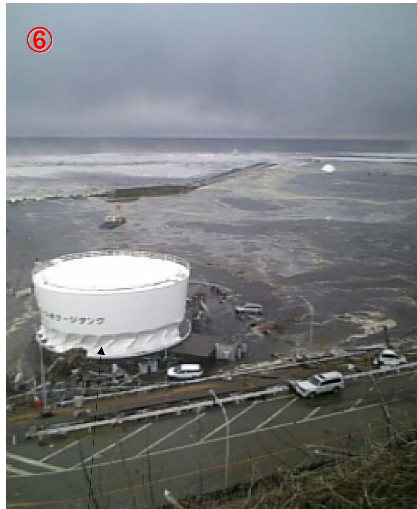
The entire body of the giant surge tank has been contorted as if a PET bottle is wrenched
