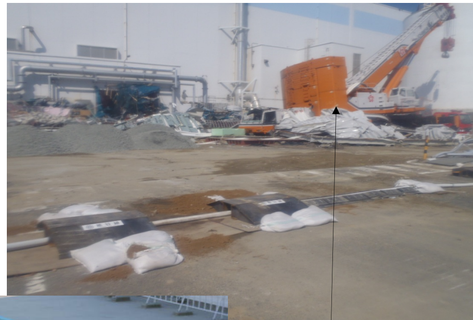
Crane vehicle (45t) and debris have been drifted, and obstructed the access to the building
