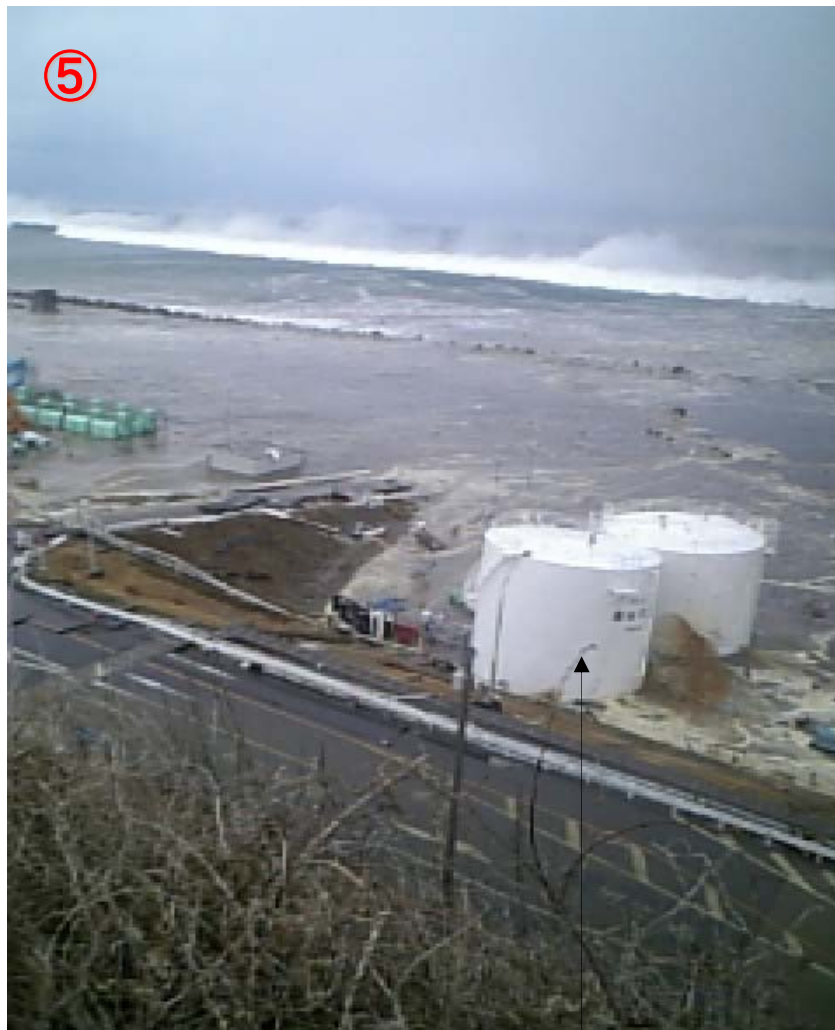
2 heavy fuel tanks have been drifted, and pushed up towards the roadside.
