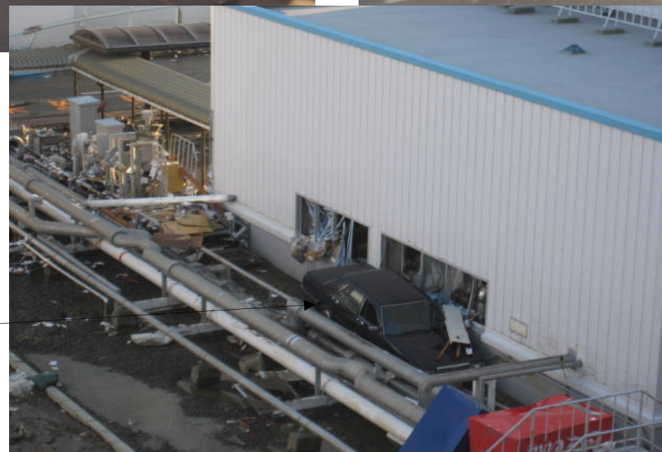
Crane vehicle (45t) and debris have been drifted, and obstructed the access to the building
